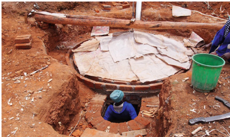
Fig. 5.15 A below-ground biogas digester being constructed in Malawi (courtesy P. Dauenhauer)
