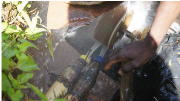
Fig. 6.27 An improvised hydroturbine in Malawi. Notice the use of plastic beverage bottles for nozzles (courtesy P. Dauenhauer)
