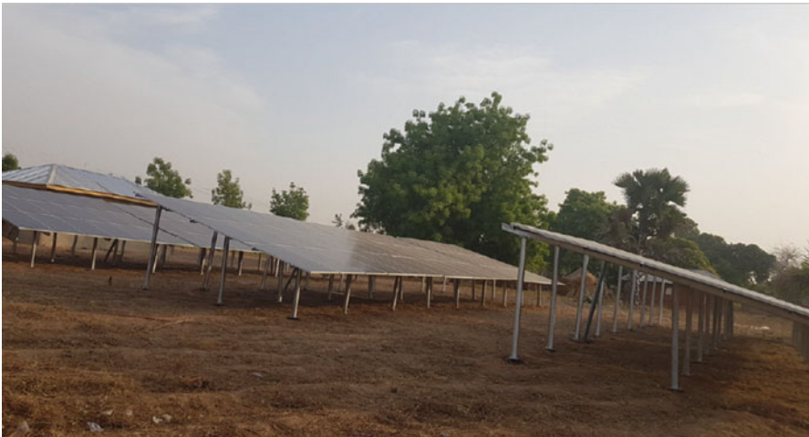
Fig. 11.11 PV modules like these for a mini-grid in Angwan Rina, Nigeria, are often mounted on a rack to obtain the desired tilt (courtesy of GVE Projects)
