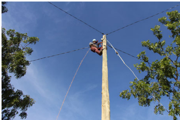
Fig. 12.10 An overhead low-voltage distribution line being installed (courtesy of PowerGen)
