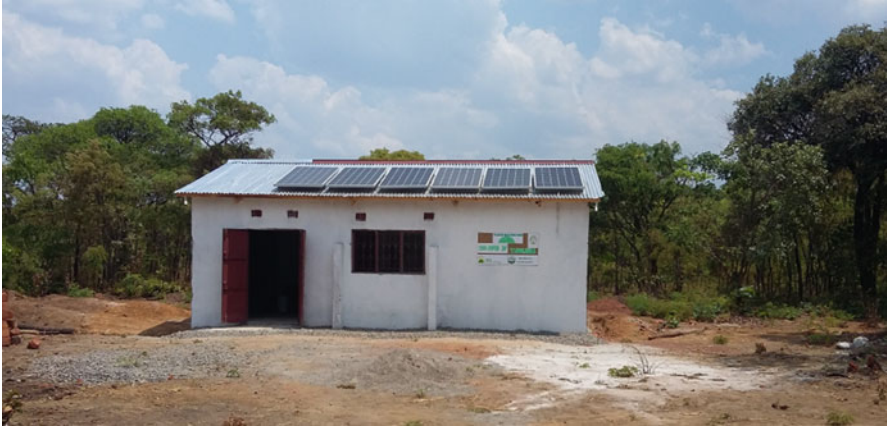
Fig. 12.25 The energy kiosk in Filibaba, Zambia (courtesy of KiloWatts for Humanity)
