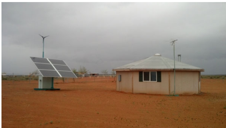
Fig. 1.16 An off-grid system in the Navajo Reservation in the United States (courtesy D. Terry, Navajo Tribal Utility Authority)
