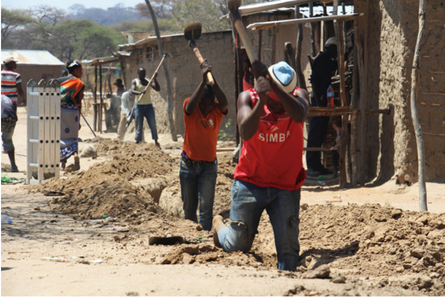
Fig. 12.9 Trenches being dug for underground distribution (courtesy of PowerGen)
