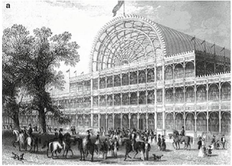
Fig. 2.10 Examples of structures made of iron trusses. (a) Crystal Palace. (b) Eiffel Tower. (c) Saint Pancras station
