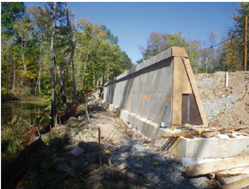
Fig. 8.4 Cantilever wall construction
