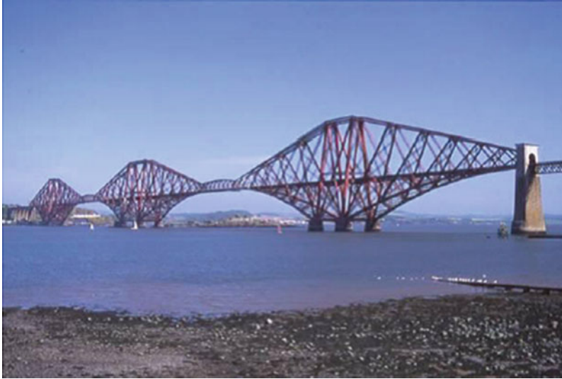
Fig. 2.12 Example of early steel bridges—Firth of Forth Bridge, Scotland
