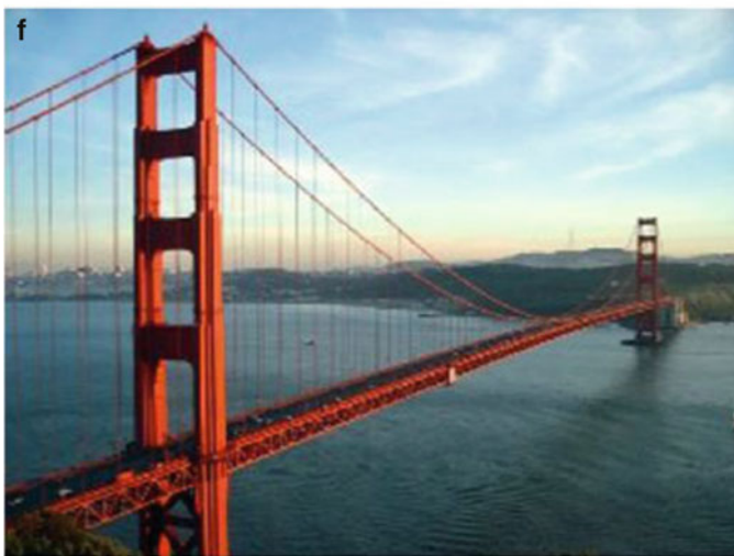
Cable-girder system (suspension bridge)
