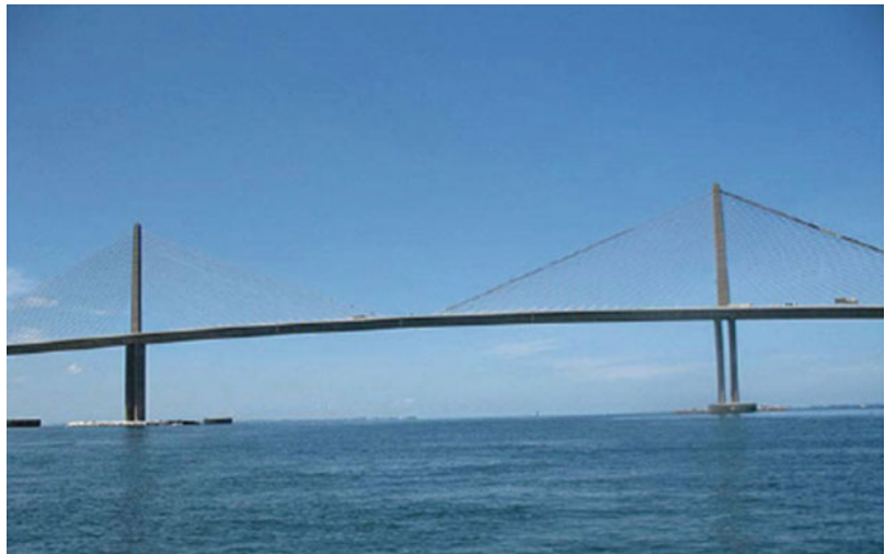
Fig. 13.34 Typical cable-stayed scheme
