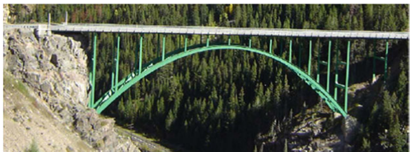
Fig. 13.27 Two-hinged arch bridge
