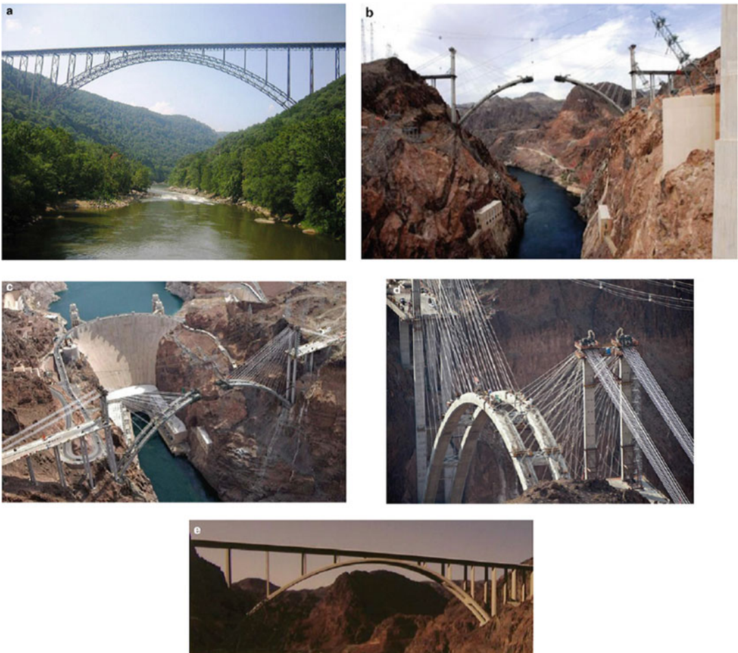
Fig. 6.9 Modern Arch Bridges in the USA. (a) New Gorge Arch, West Virginia. (b) Hoover Dam Bypass—under construction. (c) Hoover Dam Bypass—under construction. (d) Hoover Dam Bypass—under construction. (e) Hoover Dam Bypass—completed
