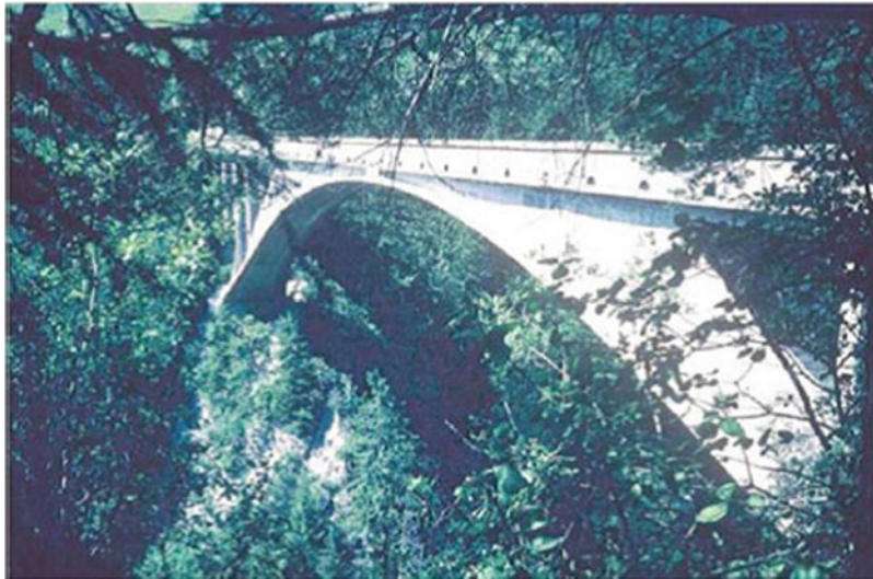
Fig. 6.8 Salginatobel Bridge, Switzerland
