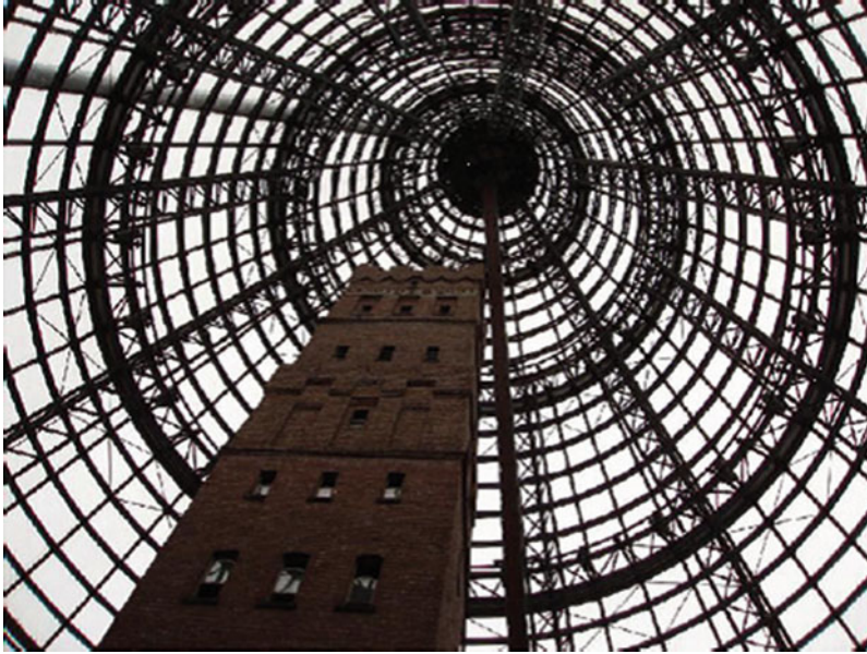
Fig. 2.13 Three-dimensional truss roof system
