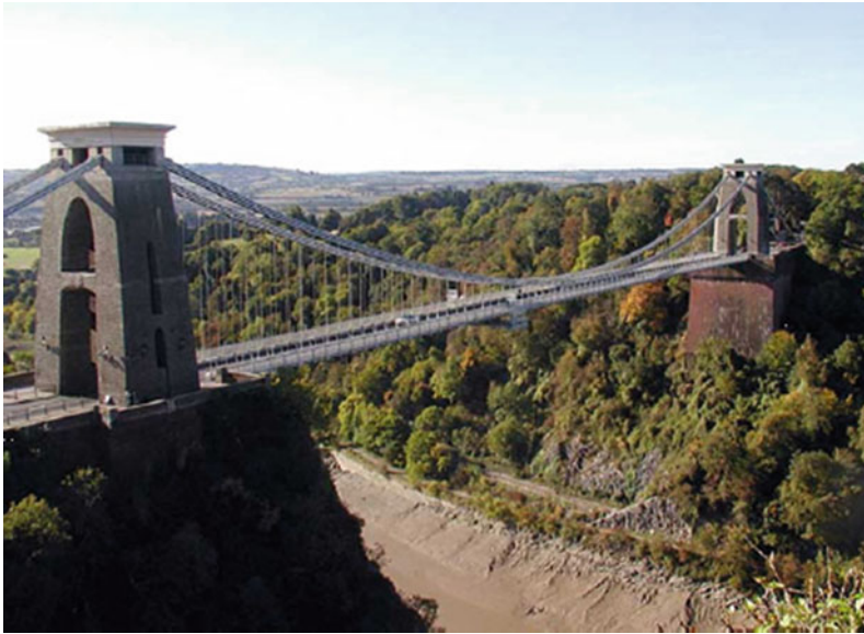
Fig. 5.1 Clifton Suspension Bridge, England
