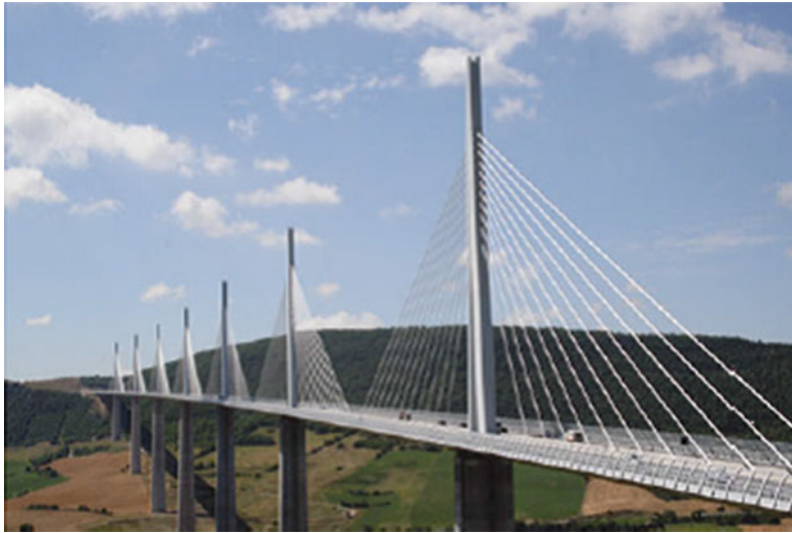
Fig. 5.21 Millau Viaduct Bridge in France
