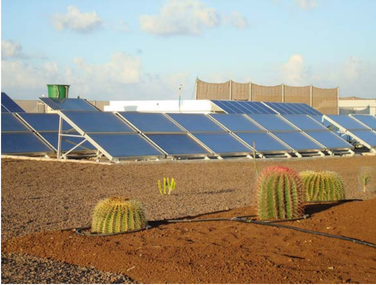
Fig. 7.13 Collector field of the Two-loop system in Grand Canary, Spain
