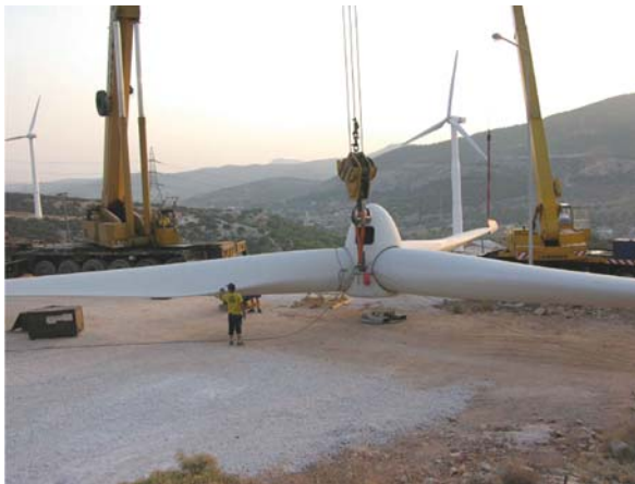
Fig. 9.3 Erection of the rotor of a W/T Source: CRES
