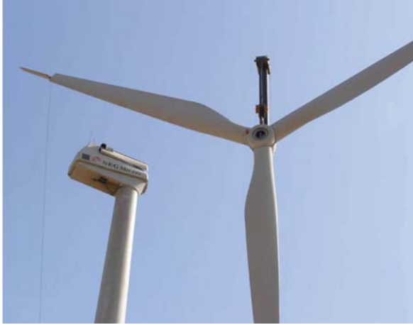
Fig. 9.6 Erection of a W/T Source: CRES
