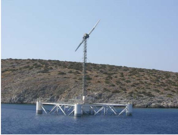
Fig. 9.23 View of the offshore Wind/RO unit in Irakleia island, Greece
