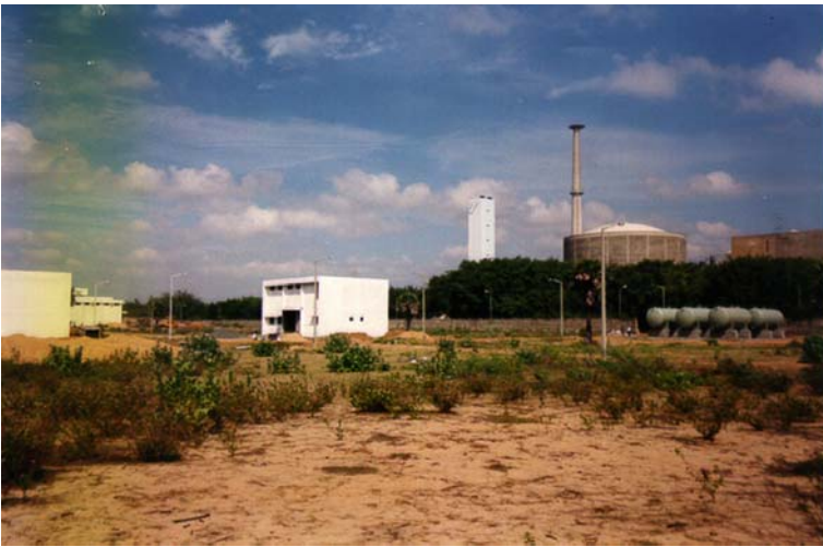
Fig. 5.5 Hybrid (MSF/RO) plant, Kalpakkam, India
