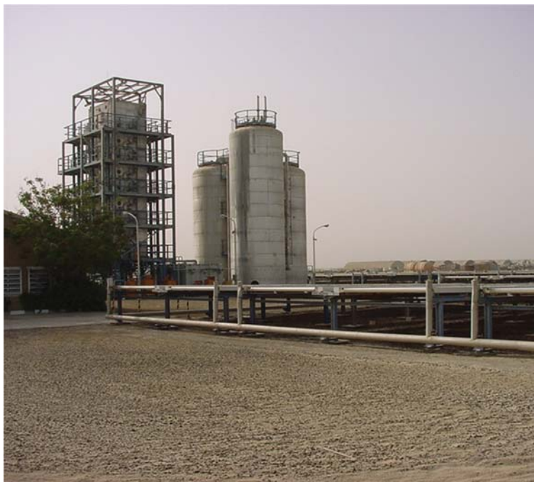
Fig. 6.14 The Abu Dhabi solar desalination plant
