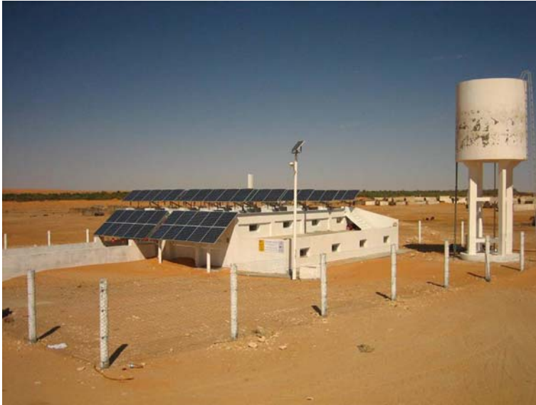
Fig. 10.5 The building housing the RO system, the PV and the water storage tank of the PV/RO system in Tunisia
