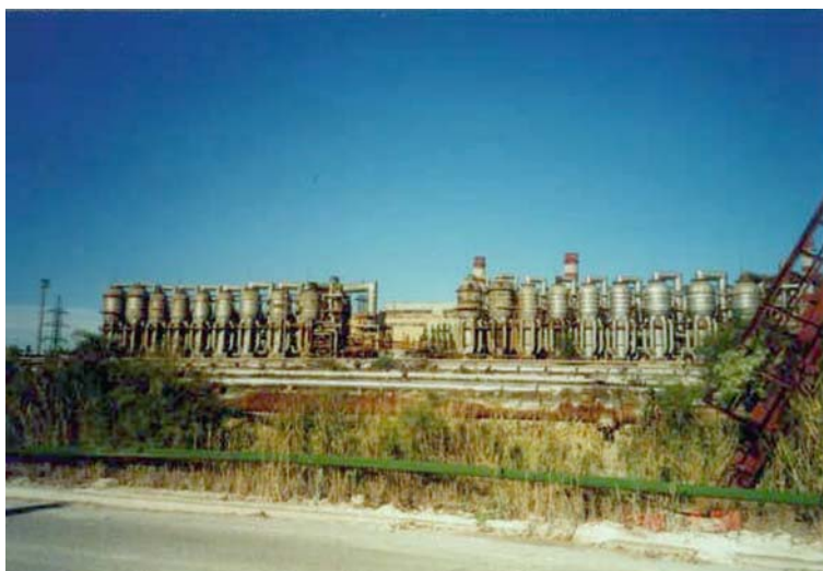
Fig. 5.3 Evaporators, Aktau, Kazakhstan
